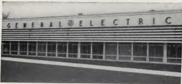
L-6: Fabricated porcelain enameled iron letters, block style, with trademark emblem also in porcelain enamel, two colors.
